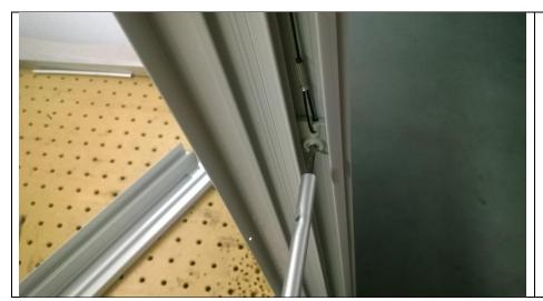
Tension the cords with the cord tensioner and an Allen key.
